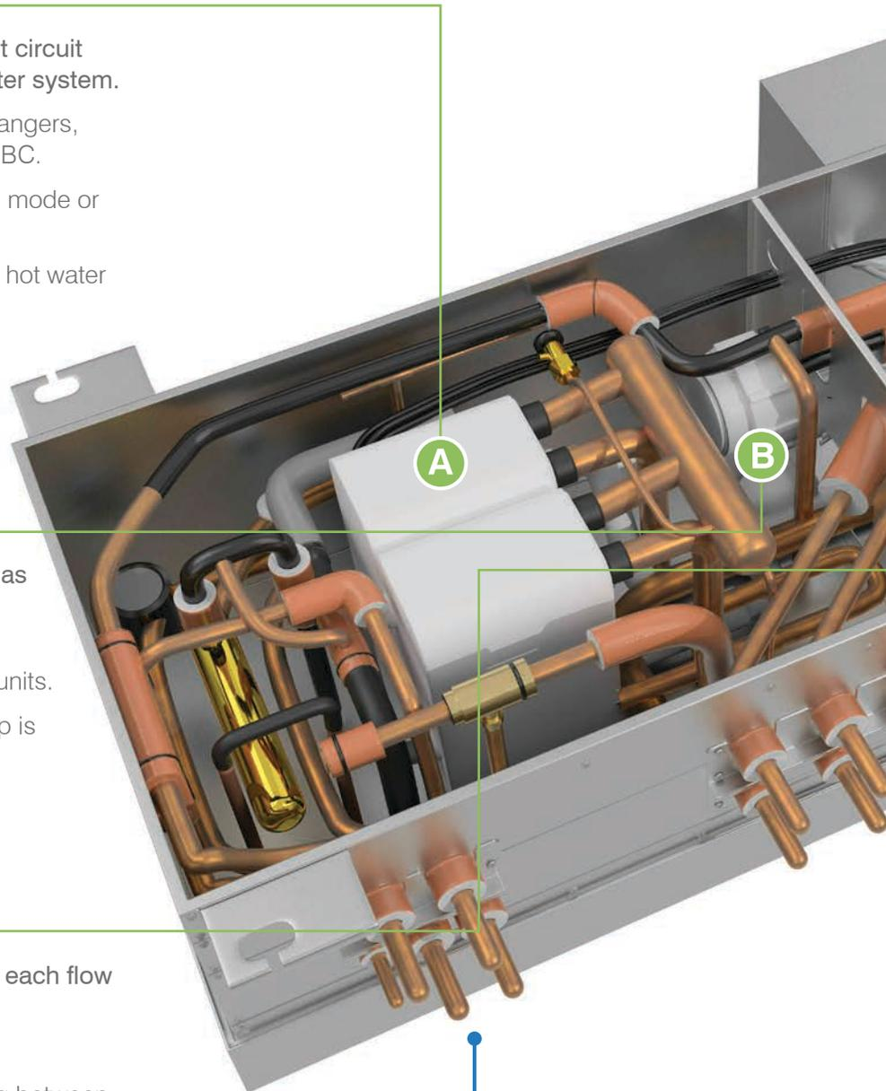
Refrigerant pipes to outdoor unit, expansion tank (field supplied) and water filling loop (field supplied)
