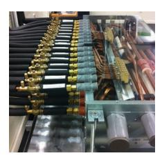
Mitsubishi Electric branch controller fitted with refrigeration ball valves for ease of maintenance and fit out flexibility.
